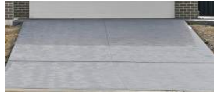
Concrete broom finish (Up to 50 sqm)
